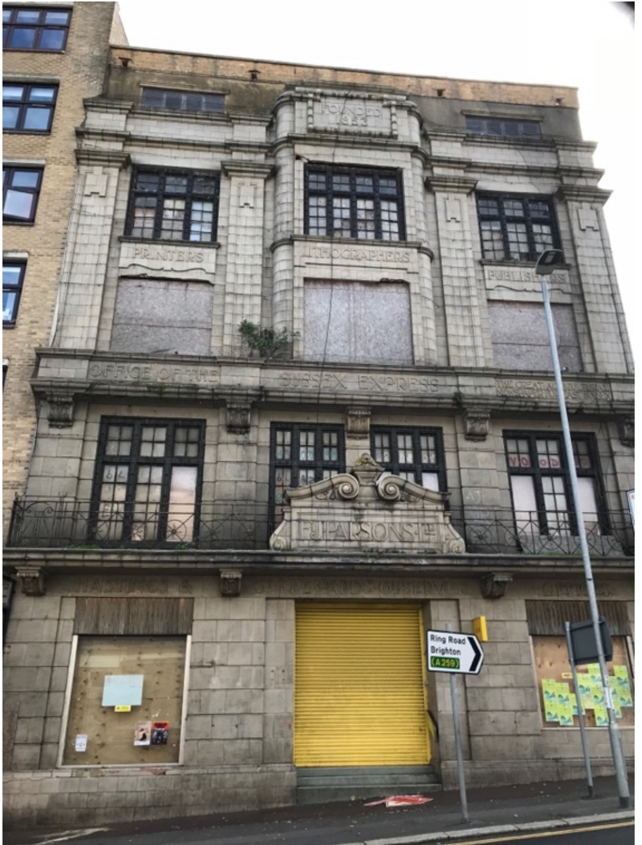
The Observer Building, 53 Cambridge Road
